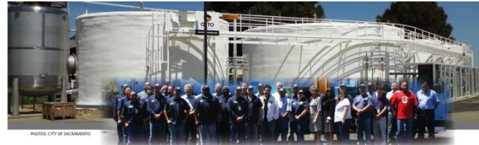
The City of Sacramento's fleet department (inset) has reduced gasoline consumption by 10 percent since 2011 and increased the use of compressed natural gas (CNG), due to the Sacramento BioDigester (above), an anaerobic digestion system that converts 25 tons of food waste into different forms of renewable energy.
